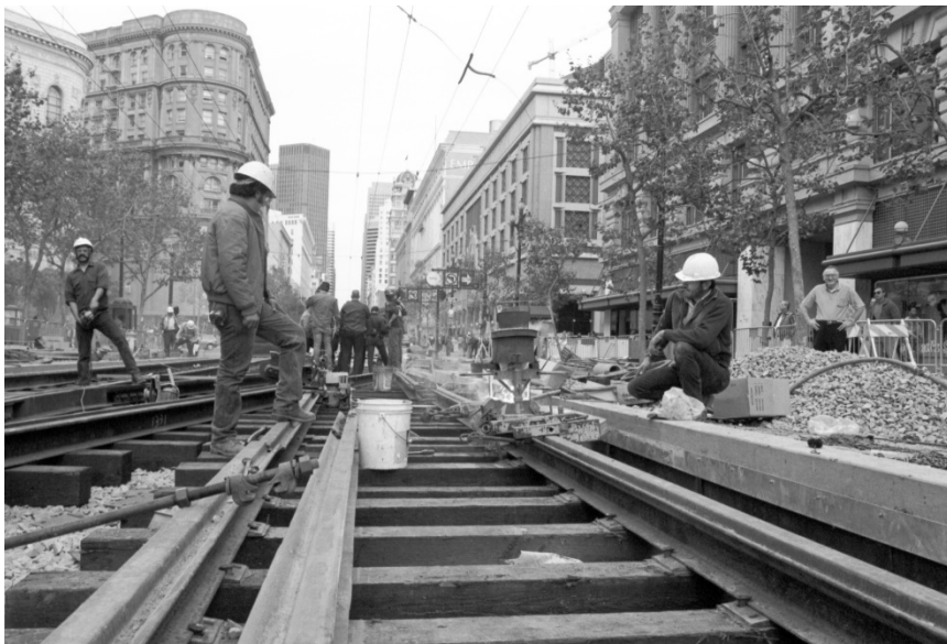
Installation of tie & ballast tracks (1988)
