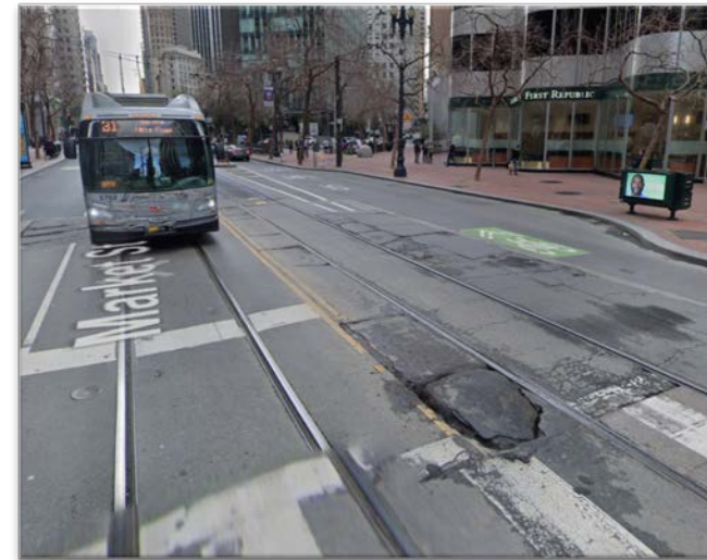
Existing pavement conditions
