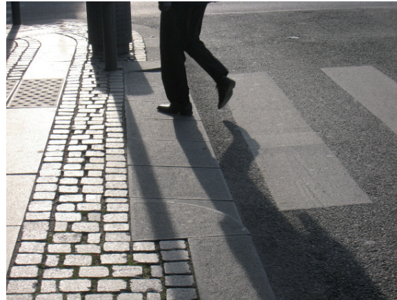
Smooth transitions ensure access for all and contribute to a comfortable walking experience. Copenhagen, Denmark
