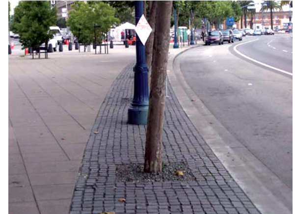
Permeable paving suspended above structural soil allows for stormwater filtration and root development.
