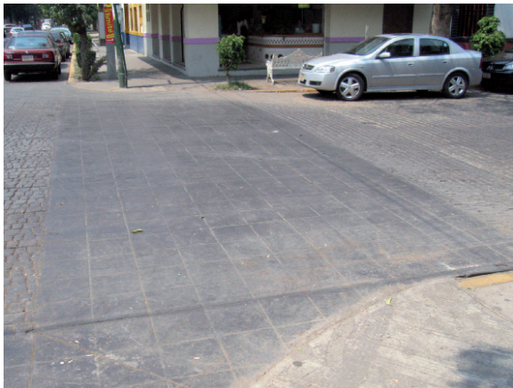
Change of material at intersection. Mexico City, Mexico
