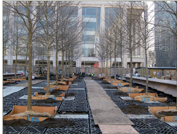
Lincoln Center Plaza suspended pavement structure during construction. New York, NY
