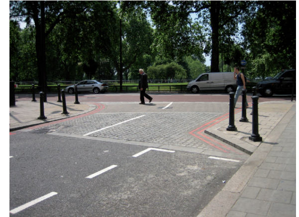
Narrowing the street and a change of materials make it easier for pedestrians to cross the side streets and drivers are made aware of pedestrians. London U.K.
