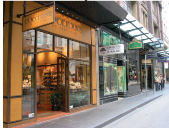
Active and attractive ground floors integrate many units, many doors, and a high level of transparency. Melbourne, Australia
