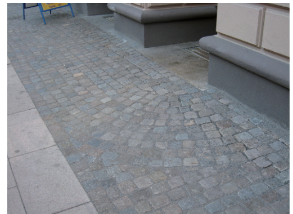
No differences in levels providing easy access to ground floor uses. Ystad, Sweden
